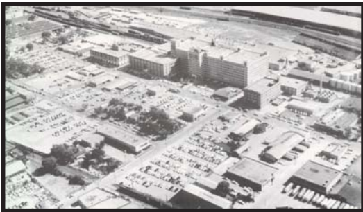
The old Sears Catalog Warehouse and adjacent rail yards in the late 1950s.
